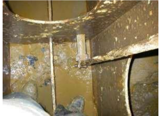
Mud and sediments can contain MIC
