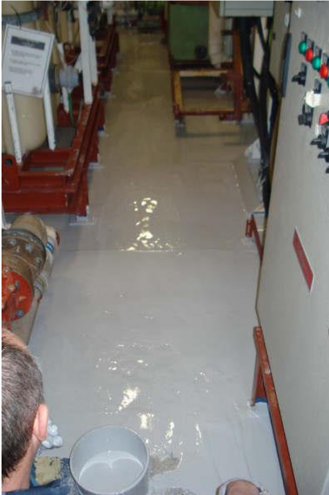
Note: Thick section applied in 1 coat
