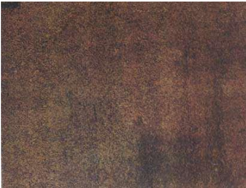
Scraping and wire-brushing
